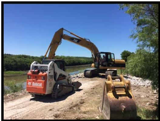
On June 27, 2015, the dike separating the Marsh from Lake Erie was heavily damaged by a nor'easter that pushed Lake Erie up and over the dike; damaging more than 5,400 linear feet of the dike, and 1,500 linear feet was severely damaged. The members of the 200 RHS filled in the most severely damaged sections with over 600 tons of type “D” rock to stop the dike erosion.
