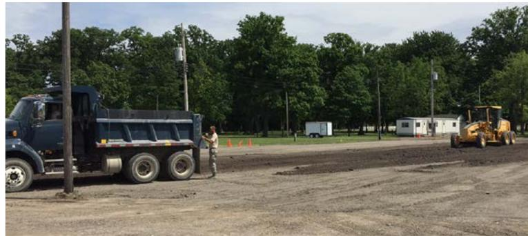
The main parking, roughly 37,400 square feet, consisted of poorly graded asphalt, which resulted in water penetration to the sub-grade and ultimately failure in multiple areas. Creating an eyesore and hazard with standing water, and ice in the winter. The RED HORSE team removed the
