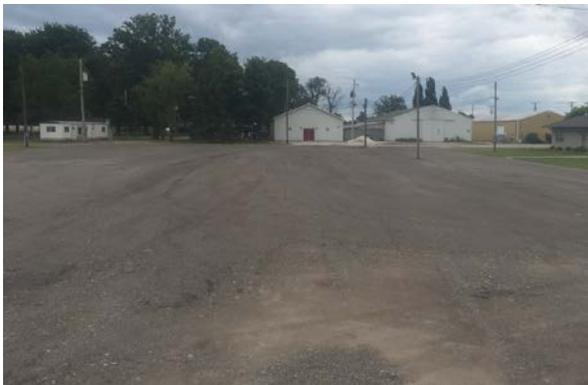
existing pavement and stabilized the sub-grade. Then, using the asphalt millings provided by the county, the airmen were able to spread, grade, and slope to implement a compaction plan that directed water shed and ensured proper drainage. In addition the airmen were able to utilize these millings to repair other vehicle area at the fairgrounds.
